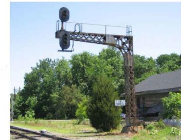
6. CANTILEVERED SIGNAL TRUSS
